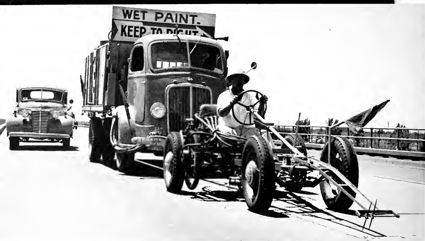
View of broken traffic line striping equipment in operation on State highway
